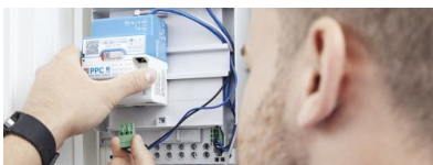
Installation eines Smart Meter Gateways. Quelle: Voltaris
