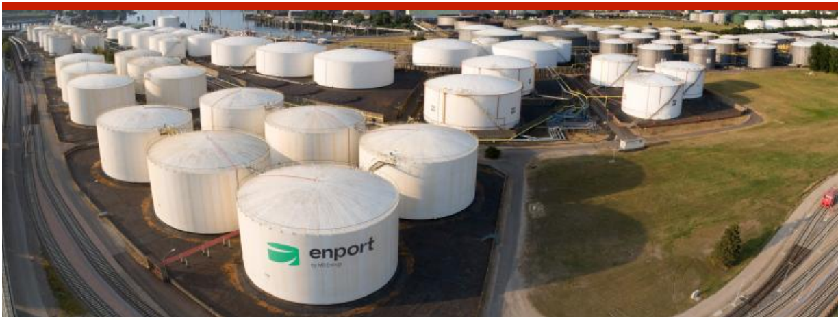
Tanklager "Blumensand" in Hamburg. Quelle: MB Energy
